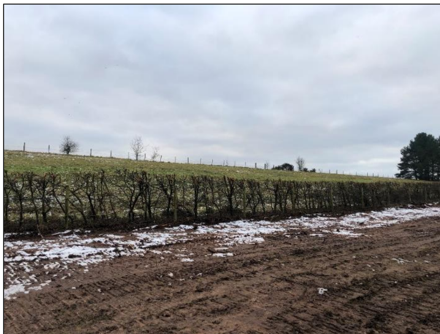
Figure B: Photograph of the norther lagoon embankment
