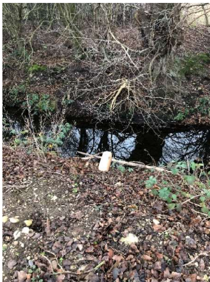
Example of current outfall to tributary of the River Idle
